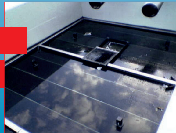
Customized Skimmer for floating roof in tanks and vessels
